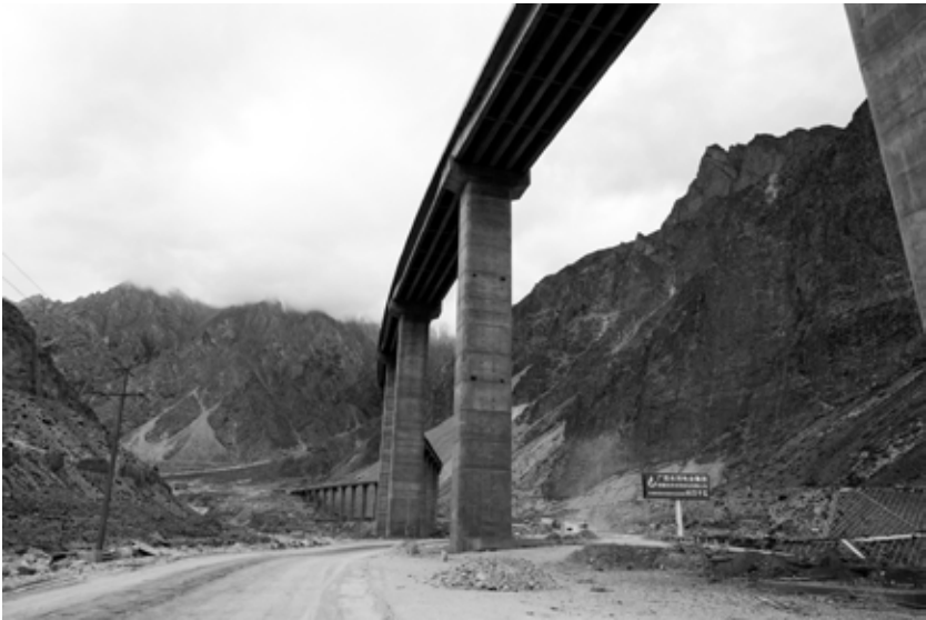
Figure 15: Suspension bridges on the new KKH in the Gez Canyon (picture by the author, 2016)
