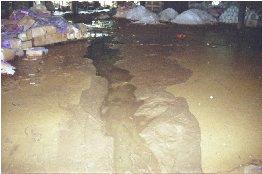
Water streams through the heaps of asbestos © Private collection Ronald Geval
