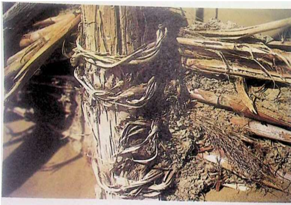
98. Niya: it is impressive to note how the walls were literally tied to the wooden poles by means of a kind of raffia rope.
