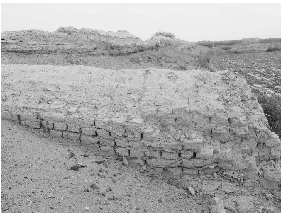
Figure 2.3. The north-side wall of Toupu (Tougongbao) (Photo: Onuma, 2015)
